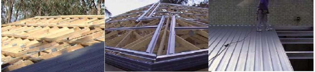
Fixes to Timber Battens
